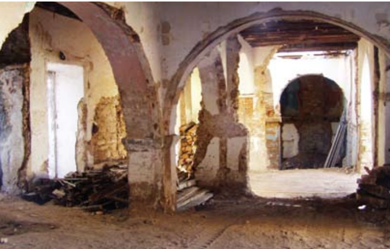
✂ Estrutura de arcaria original, na ala nascente do Colégio, AG, 2009 Structure of original arcade in the east wing of the College, AG, 2009
