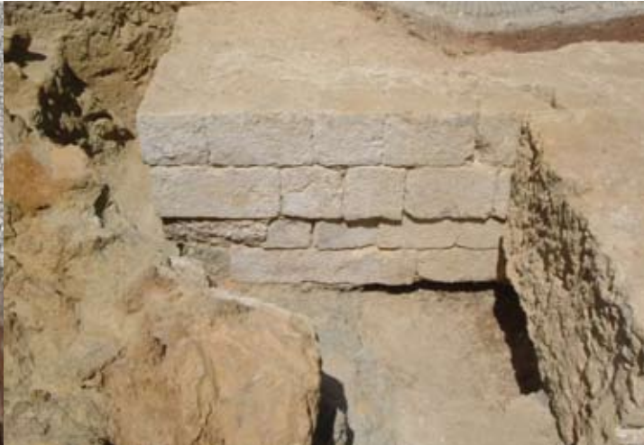
✕ Canto oeste do embasamento da Torre do Castelo de Coimbra, após desconstrução do contraforte (Sondagem A), SF, 2008 West corner of the foundation of the Keep of the Castle of Coimbra after deconstruction of the buttress (Survey A), SF, 2008
