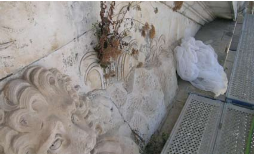
☒ Limpeza após aplicação de biocida na fachada sul, GCU, 2009 Cleaning after application of biocide in the south façade, GCU, 2009
