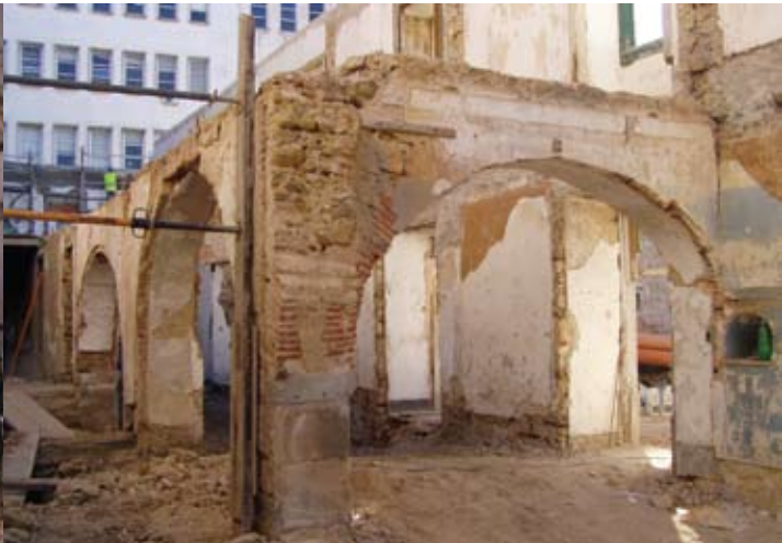
✂ Pormenor da estrutura em arcaria original, no rés-do-chão do Colégio, AG, 2009 Detail of the structure of original arcade on the ground floor of the College, AG, 2009
