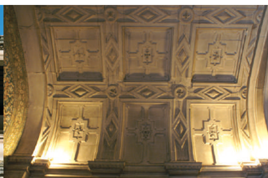
☑ Pormenor da abóbada que suporta o coro-alto, RF, 2006 Detail of the vault supporting the upper choir, RF 2006
