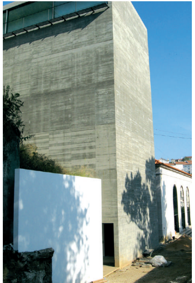
☑ Fachadas sudoeste e sudeste do edifício, após a intervenção, SA, 2008 Southwest and southeast façades of the building after intervention, SA, 2008
