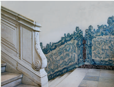
☑ Pormenor da escada de aparato, MR, 2009 Detail of grand staircase, MR, 2009
