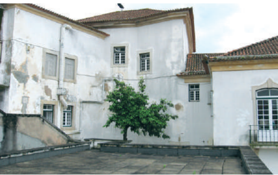
☑ Fachada norte, CM, 2008 North façade, CM, 2008
