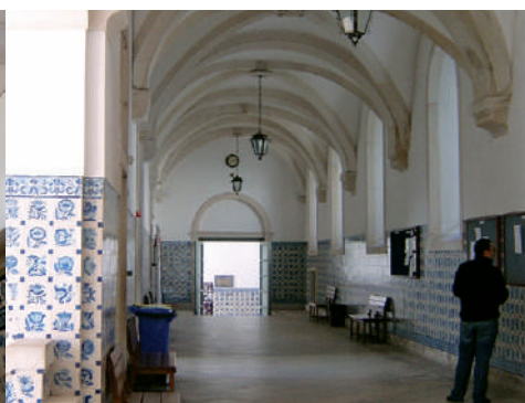
☑ Corredor abobadado do piso térreo, SP, 2006 Vaulted corridor on the ground floor, SP, 2006
